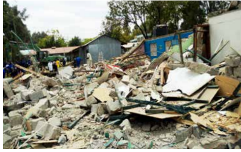
Demolished MCH building
