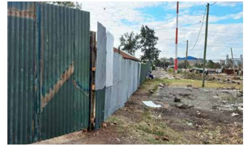
Improvised fence after demolition
