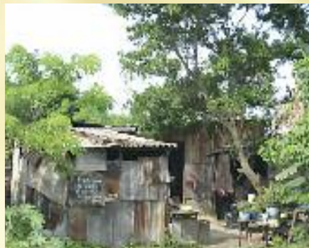
Homes in rural areas are often constructed with poor materials.
