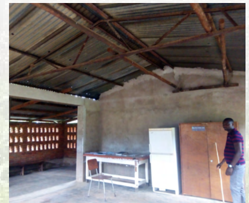
Preparing the new building
