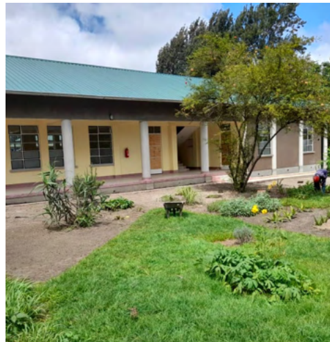
A view of the new classrooms
