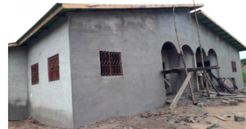
The new doctor's house - roofed and plastered
