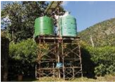
The solar water pump ensures services at the health centre.
