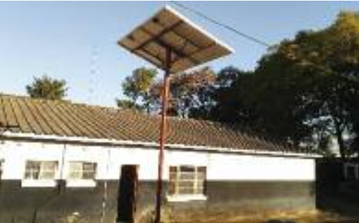
Solar panels installed at Kasina Health Centre
