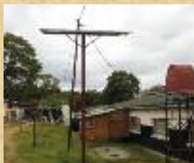
Solar power outside the maternity ward
