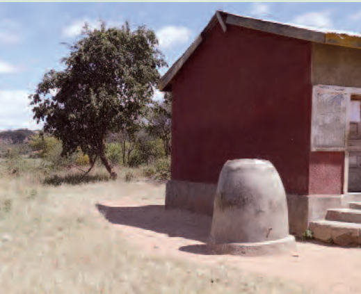
A handmade water storage tank
