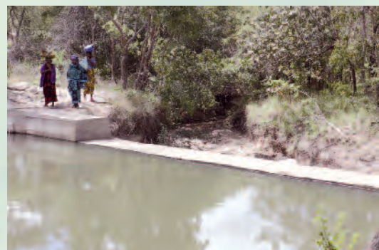
Water building up behind the Matangarimo dam
