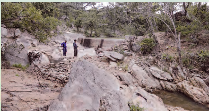
Viewing the completed dam
