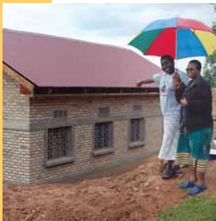
Sisters Goretta and Angelina watched excitedly as the new health outpost was being constructed.
