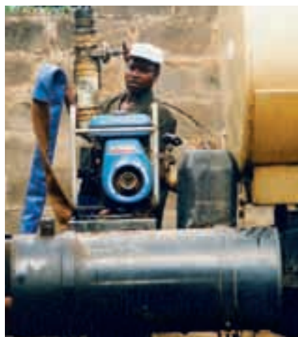
Submersible pump is installed at Abakaliki.
