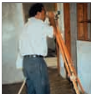
Civil Engineer Thomas Shaibu checking levels
