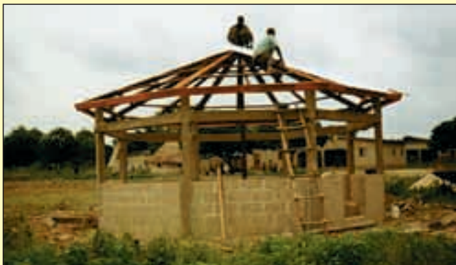
Nutrition Unit under construction
