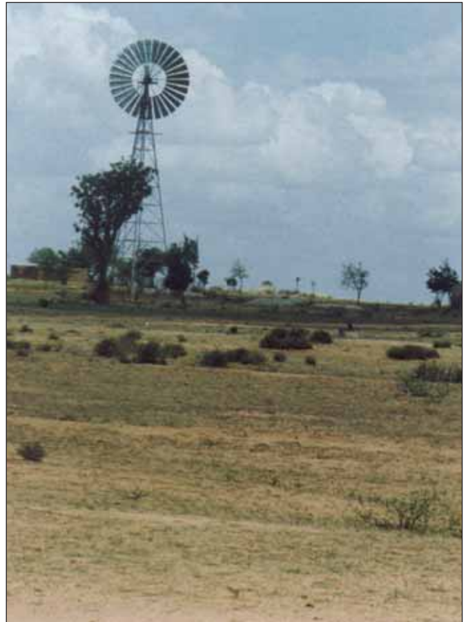
The hospital's water supply is pumped by windpower from a borehole.
